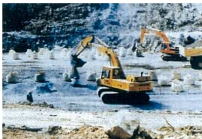
Soft ground improvement construction.
