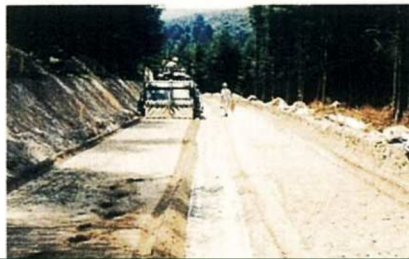
Constructions of forestry roads.
