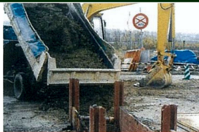
Backfilling of plumbing works.
