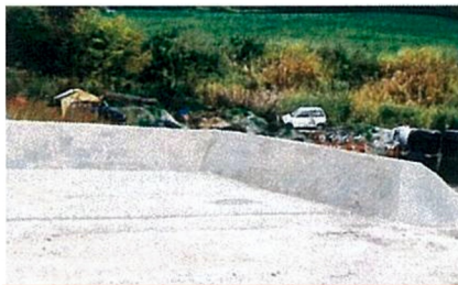
Constructions of barnyard manure reservoirs.
