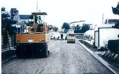
Constructions of base courses and sub base courses of road.
