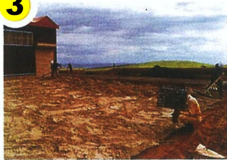
Spreading-out of the STEIN-R equally on the sites out of packages.
