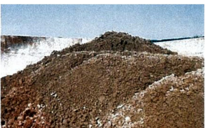
Hardening of cover soils and embankments.
