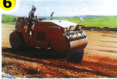
Rolling compaction. Rolling should be executed as soon as the leveling-off work is finished.
