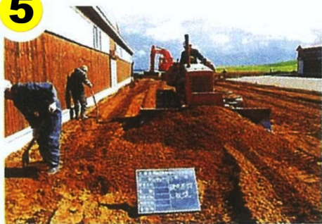
Leveling -off of the road surface.
