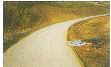
Constructions of promenade roads.
