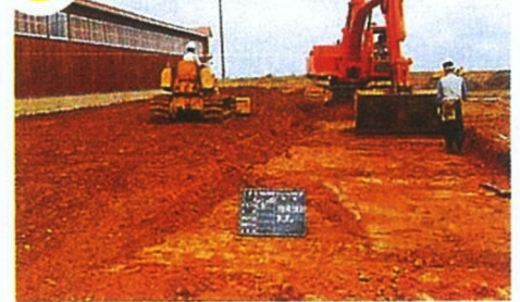
Ranking-Out of soil and eveling-off (bulldozers, rake dozers)
