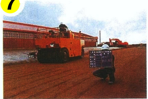
Leveling-off after rolling compaction
