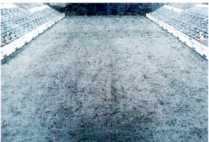
River bottom repair construction.
